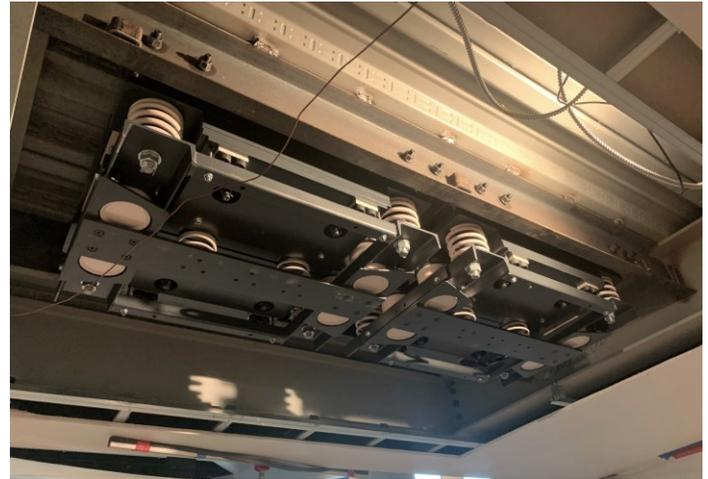
Figure 2 Installed TMDs
