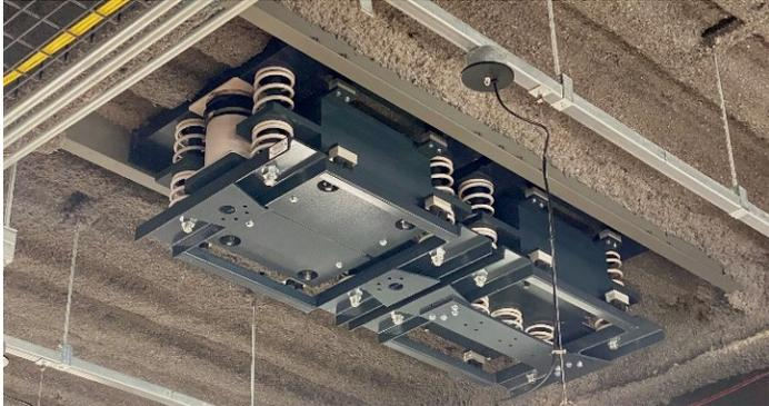
Figure 1 Two TMDs appended underneath one of bays of the floor system
