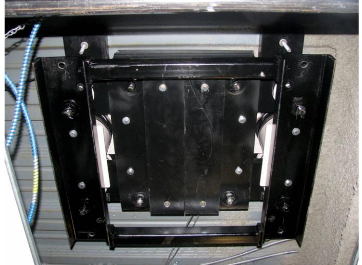
Figure 2 One of the TMDs installed underneath the floor system
