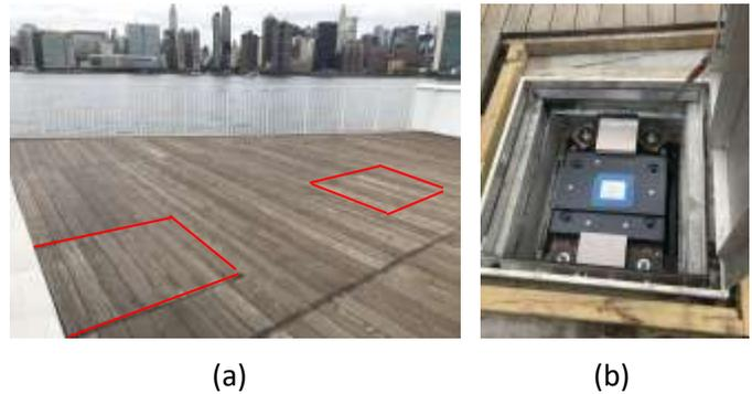
Figure 2 The locations of the TMDs (marked in red) close to the tip of the overlook (a) and one of the two TMDs placed in its cavity (b)
